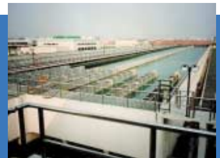
Da Chang Water Treatment Plant, Shanghai
